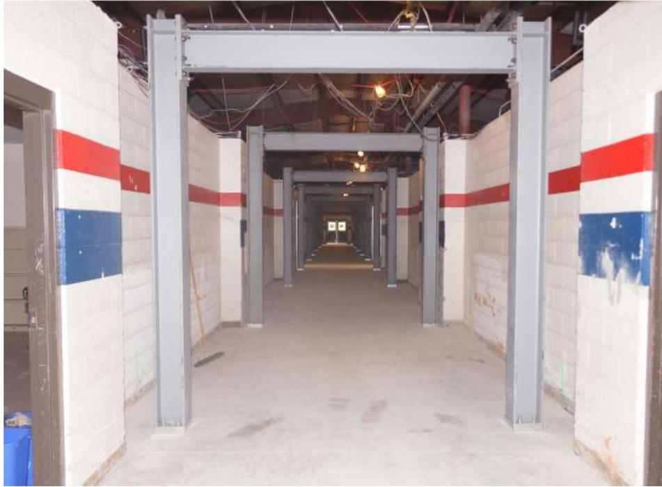
**Rigid frames resist lateral wind forces on safe room**
