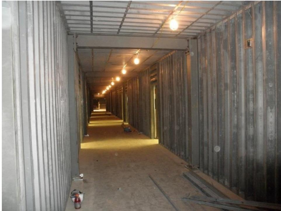
**Safe room wall and ceiling modules ready for installation of drywall**
